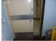
Lock is positioned too high
